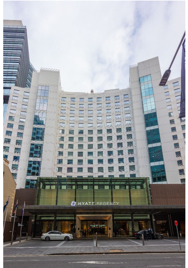
Figure 25 View of the Hyatt Regency looking west
