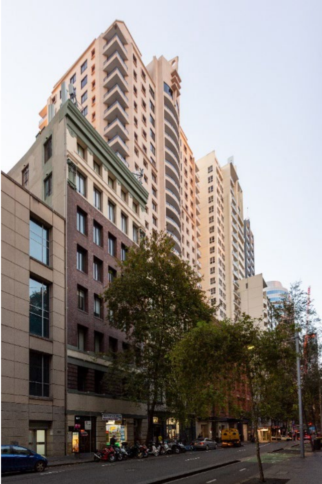
Figure 17 View along Kent Street to the north
