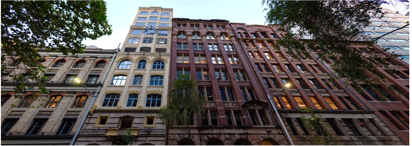
Figure 19 View to the east of the site along Kent Street looking upwards
