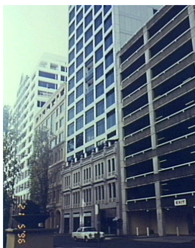
Figure 6 View of along Sussex Street (1996)
